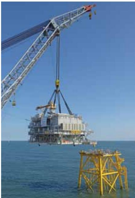
Front cover image: The installation of the Dudgeon Offshore Wind Farm offshore substation, CHPV/ Statoil. See page 5 for full story.
