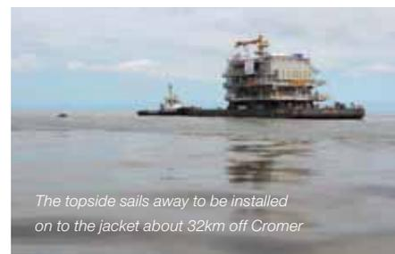
The topside sails away to be installed on to the jacket about 32km off Cromer
